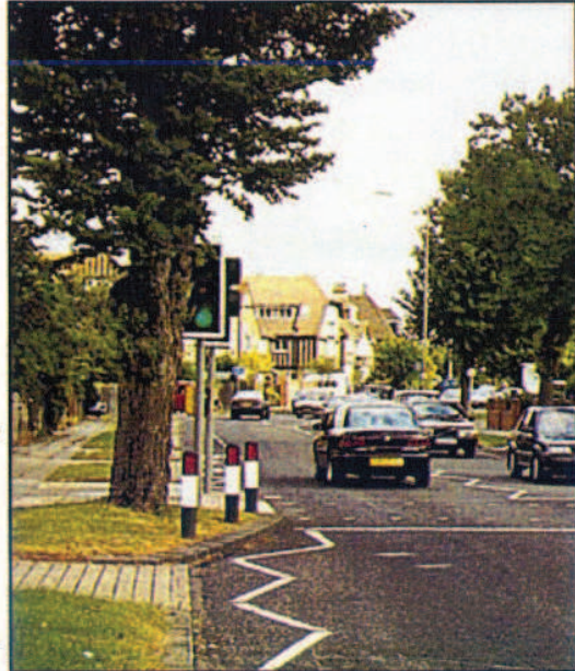
Photo of example build out at controlled crossing to improve visibility around an existing tree (taken from Local Transport Note 2/95)
